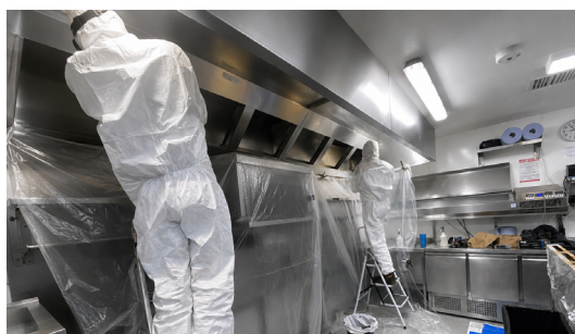
Kitchen Extract Cleaning
