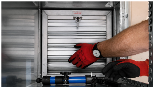
Fire Damper Remedials
