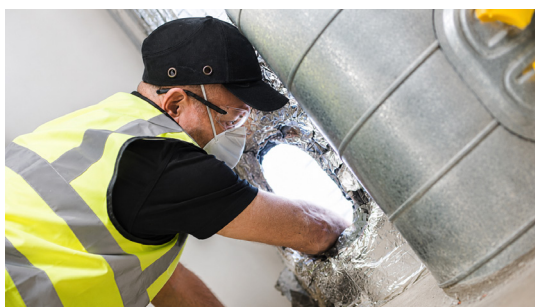
Fire Damper Testing
