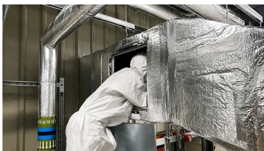
Air Duct Cleaning
